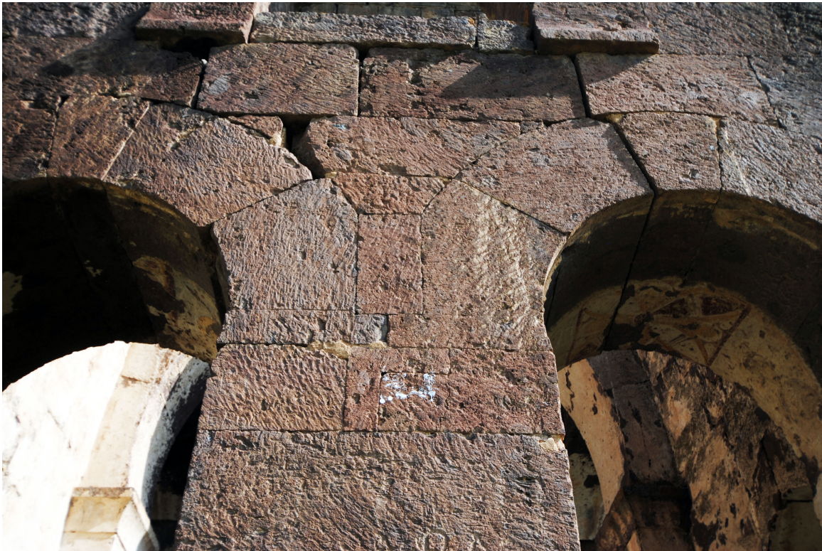
Fig. 4. Same, south façade, transept, detail of masonry construction (author)
